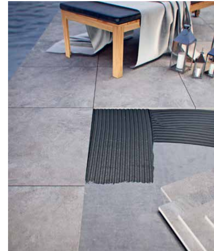
INSTALLATION OF TILES WITH THE USE OF GLUE
