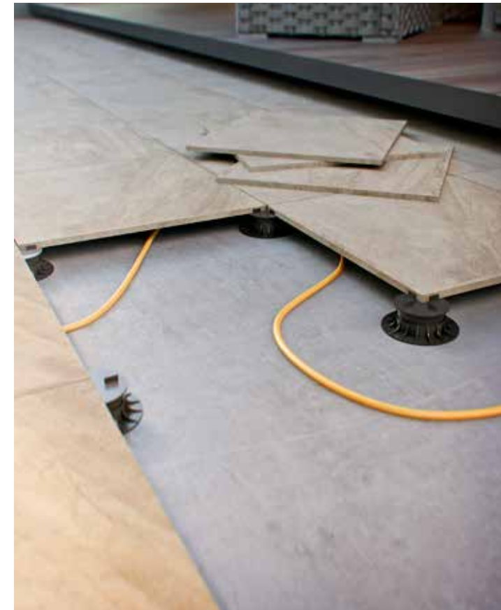
INSTALLATION OF RAISED FLOORS ON FLAT BASES
